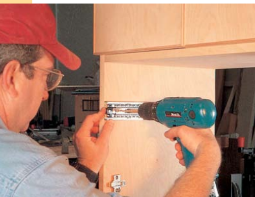
After attaching the slide to the drawer, mark the location of the cabinet part of the slide on the cabinet side. Use a framing square to run a line back from this mark and mount the slide \frac{1}{16} " back from the front of the cabinet.
