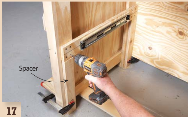
17 Mount the platform assembly's outside slide supports in the cabinet. Use spacers to level the supports and position them at the correct height.
