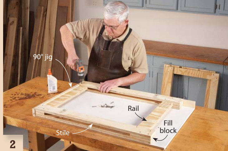
2 Assemble the cabinet's frames by stacking and gluing plywood stiles, rails and fill blocks. Use a 90° assembly jig to keep each frame square.
