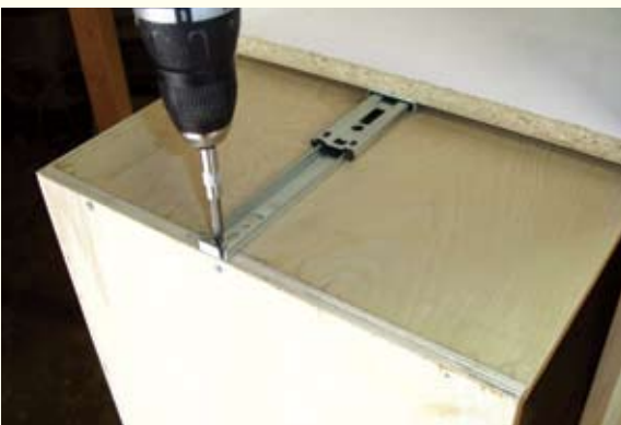
STEP FOUR I extended the drawer slide until it reached the front of the pullout, made sure the top of the shelf unit was centered in the cabinet and installed the front screw. After testing the operation of the pullout, I fully extended it and installed the back screws in the drawer slide.
