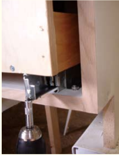
STEP TWO I set the pullout inside the cabinet on the lower pullout hardware and centered the pullout in the cabinet. The weight of the cabinet allowed me to pull the shelf unit forward without it sliding out of place on the hardware. I pulled the unit out about 5". To attach the pullout to the bottom slides, I installed the front screws first, then pulled the unit out to install the back screws.
