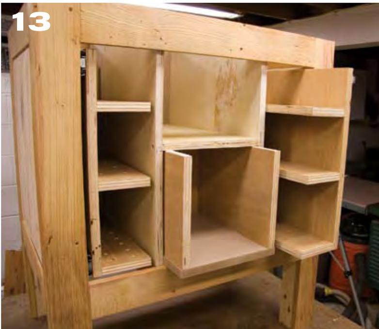
**13** Apply some paste wax to the edges of the bottom and to the top edges of the sides. The drawer should slide smoothly in and out with minimal effort. Yes, you could use mechanical slides on this drawer if you like.
