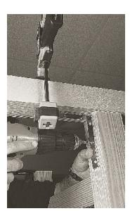
FAST AND SECURE. These 6" Lbrackets are inexpensive (about \$3 each) and install quickly – no mortising. And they are stout enough to resist wood movement forces.
