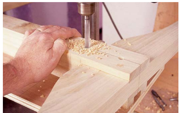
Getting the holes for the bed bolts straight is important. And the best tool for that task is the drill press. The two \frac{7}{16} " holes are located in 1\frac{1}{2} " from the top and bottom edges of the mortise.
