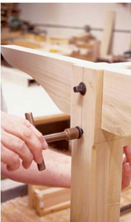
After clamping the stretcher between the legs and drilling the bed bolt holes into the stretcher I simply dropped the nut into the previously cut mortises and bolted the base together.
