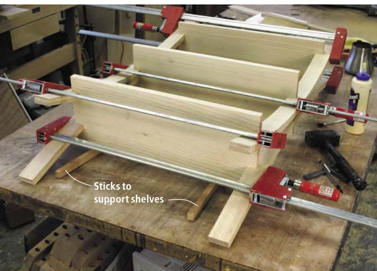
Assemble the shelves on a flat surface, making sure the ends are flat on the table. Square sticks keep the backs of the shelves in position.
