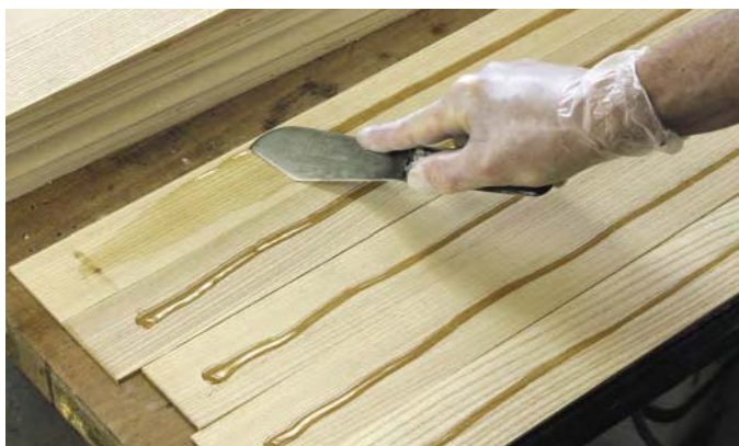
Polyurethane glue can be messy as it cures. I use a thin bead of glue and spread it out with a putty knife to avoid this.
