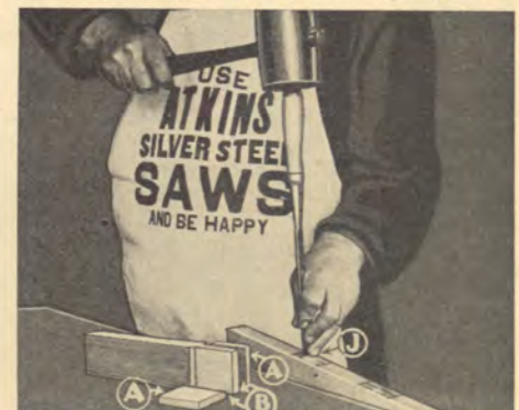
Fig. 25—Beating out mortise. Spalls A sawed from cheeks of tenon B, as shown in Fig. 14.
