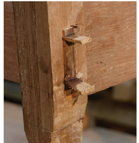
I meant to do that. The story of this joint stretches back nearly a year to the beginning of this series. The first thing I did was undercut this leg. A hasty repair was a recognition that I was in over my head with this project. As bad as this joint looks, the wedges are actually not repairs.
