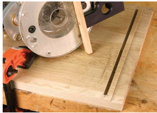
Creating the groove for the door pins to ride in is the most exacting step of the process. A plunge router with a guide fence makes it short work. Check the layout before routing.
