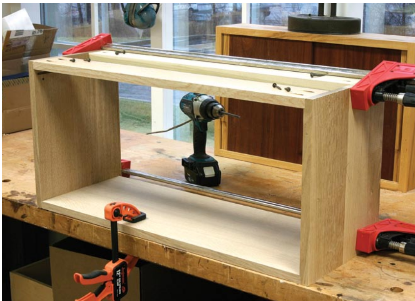
Assembling the boxes is a matter of 14 pocket screws. Clamping the box ensures that it will be square. The opening in the top is for the adjoining catch rail on a second unit.
