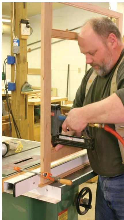
Adding a "pop." The bead is installed into the openings in the face frame. Careful measurements are key to a proper fit while glue and brads hold the bead in place.
